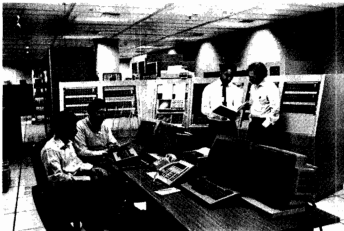
FIGURE 4: NETWORK CONTROL ROOM
